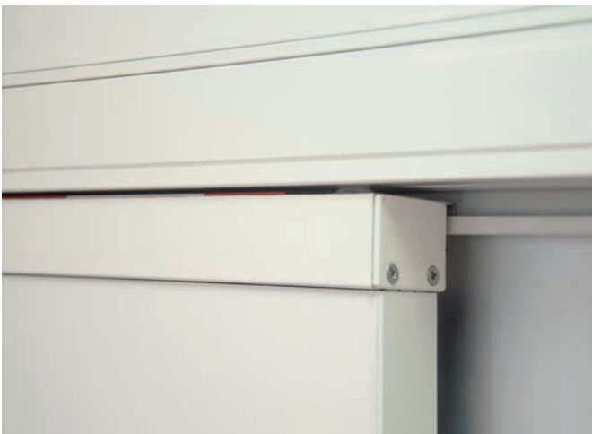
Top door leaf connected to operator
